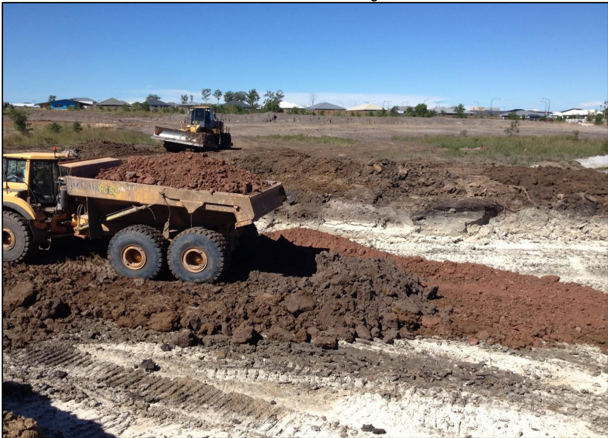
Picture 6: View of the Site during Construction
