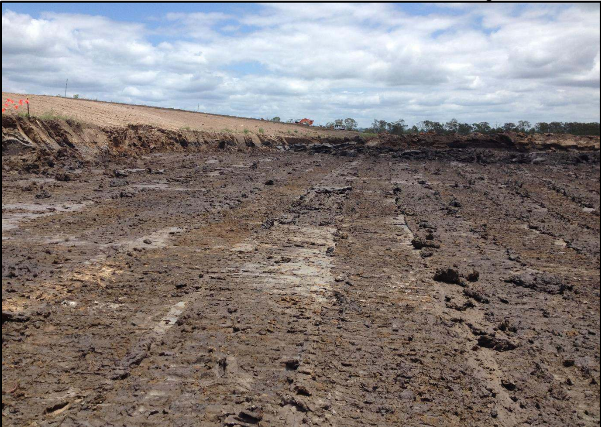
Picture 3: Excavated Surface After Removal of Unsuitable Materials in Stages 17 and 18.
