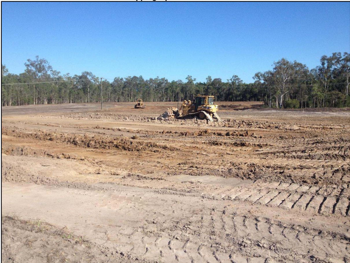
Picture 4: View of the Stripping Operations Prior to the Placement of Fill
