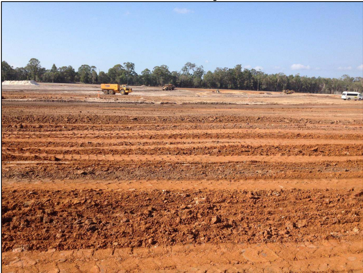
Picture 5: View of the Site during Construction
