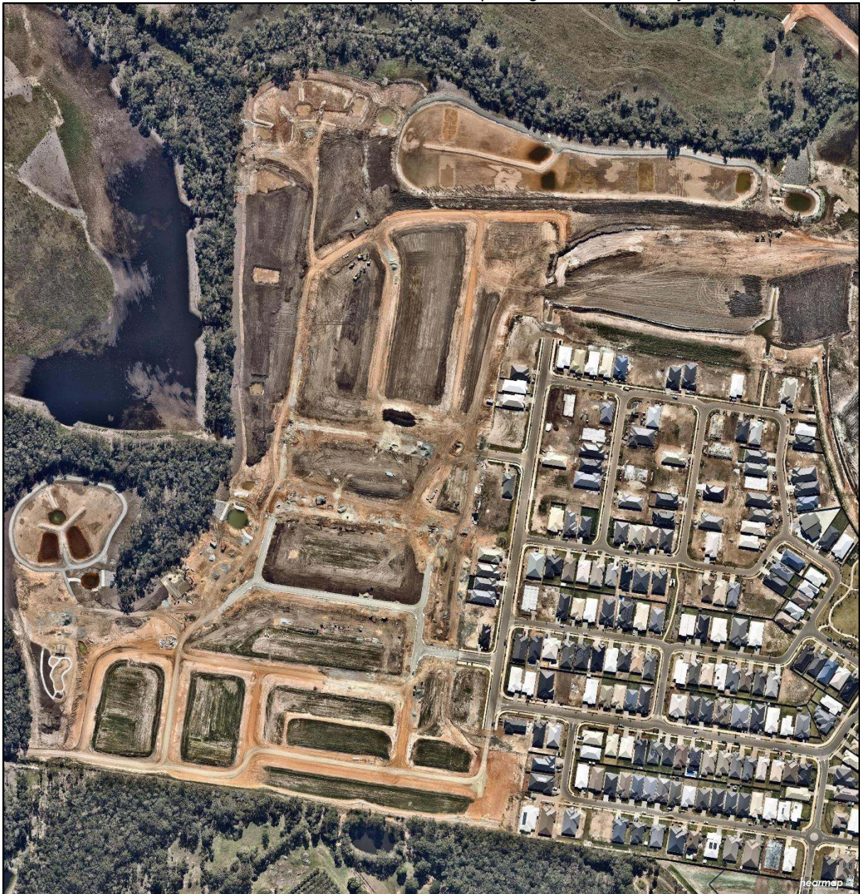
Picture 1: Aerial View of The Site (Nearmap Image, dated 22 nd July 2017)
