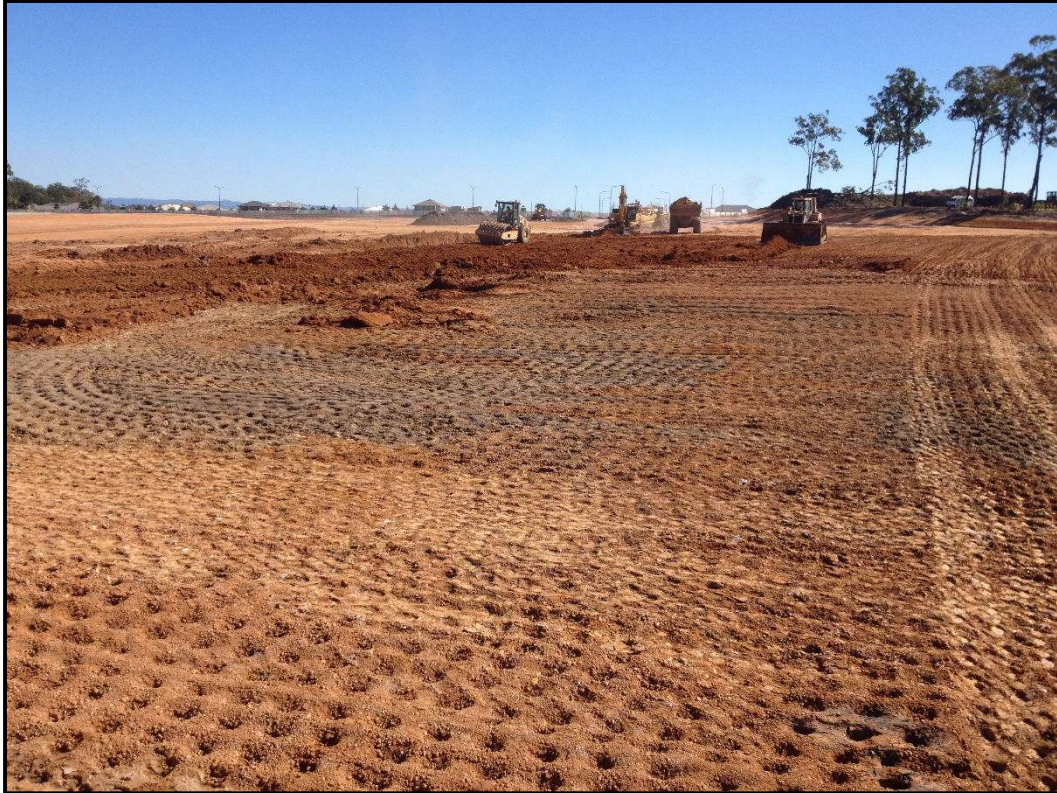
Photo 3 – View of Filling Operations
