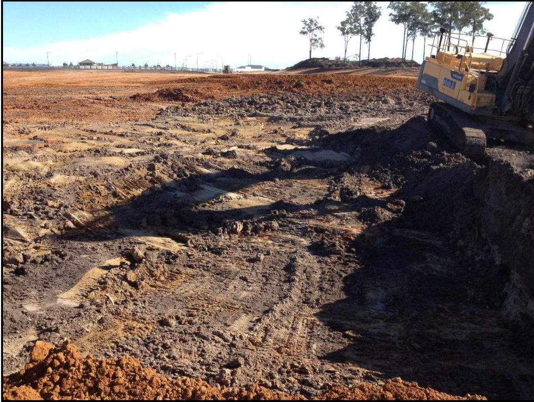
Photo 2 – View of Stripped Surface Prior to Placement of Fill
