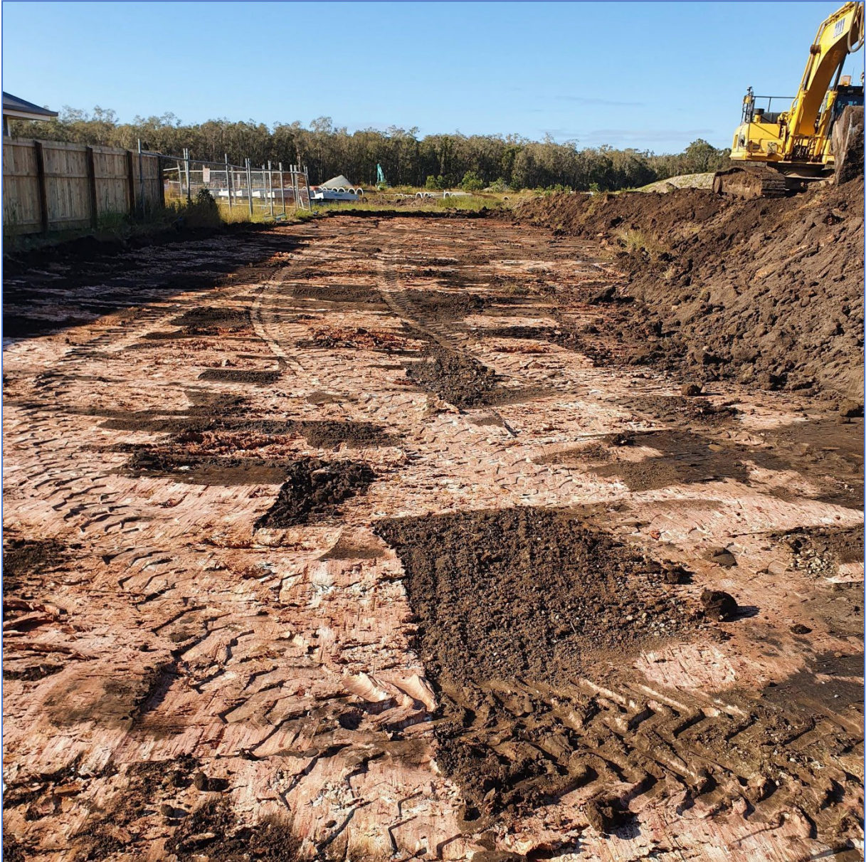
Picture 1: View of Stripped Surface
